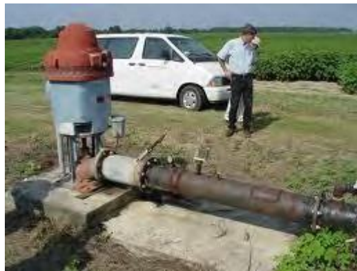
A line-shaft turbine pump is on the left. A submersible pump (right) is installed down the well from where it pumps water up a pipe to the ground surface.
