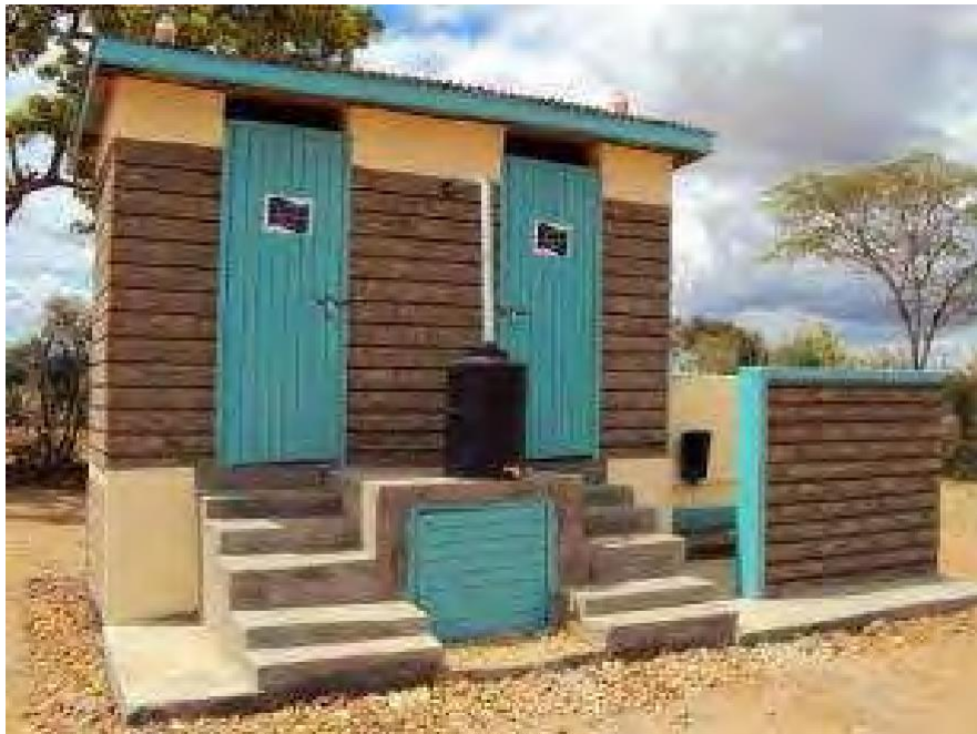
UDDT School Toilet at Nyanza, Kenya with UDDT on the left, urinal in right compartment, rainwater collector/hand washing tank.
