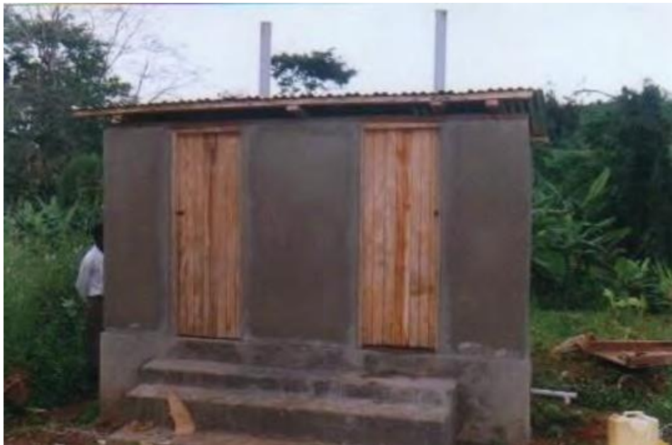
EcoSan latrine completed at Buyijja, Uganda
