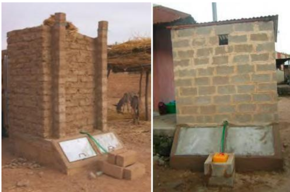
Inclined metal chamber doors inclined towards the sun to increase heat in the chambers (Source: Sswm and Crepa 2007)
