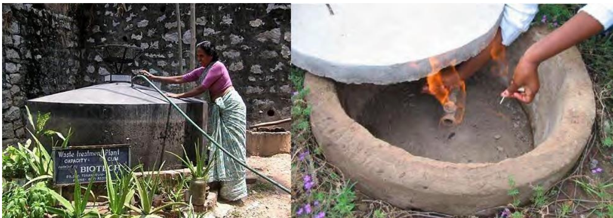
Checking the gas valve of a floating-dome biogas reactor in India (left) and lighting the biogas flame (right, Lesotho, 2006). Source: BIOTECH India (2007) and MUENCH (2008).
