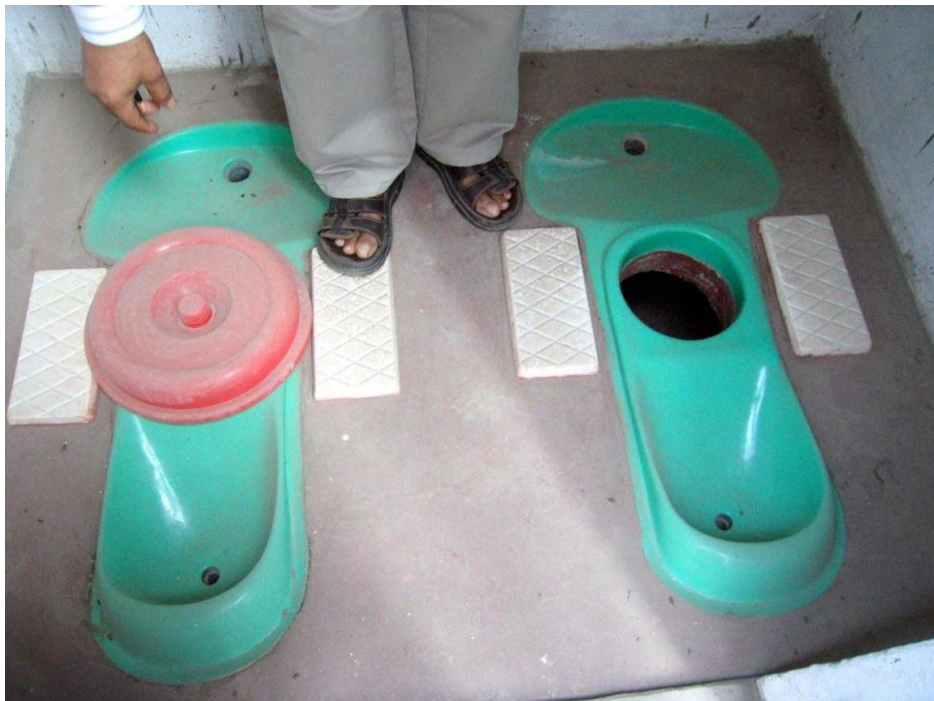
Sulabh Twin EcoSan Toilet (India) showing urine bowl (front), feces opening (center) and anal washing bowl at rear. Note separate lid to cover feces opening when second chamber is dehydrating. A second cover should also be placed over the feces opening of the chamber in use to avoid water wetting the feces during anal cleansing.
