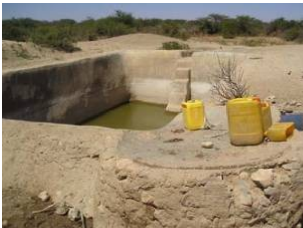
Photo 44: Berkad, the Somali name for a lined ground tank. Credit: Erik Nissen-Petersen
