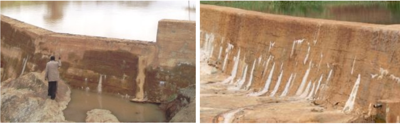
Photo 38: Monitoring leaks
