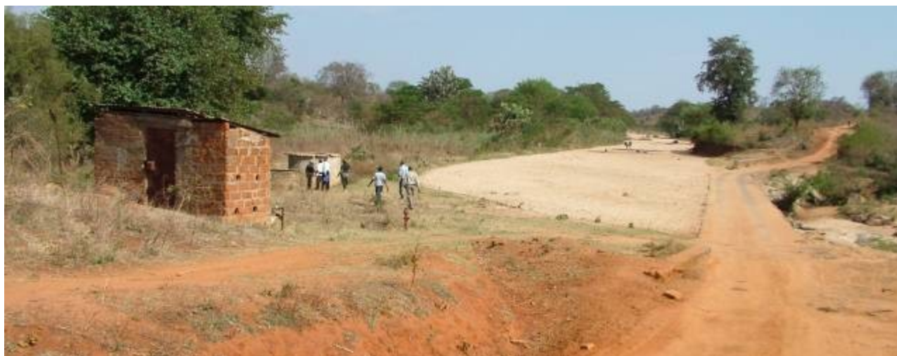
Photo 8: A sand dam road-river crossing, Makueni, Kenya.
