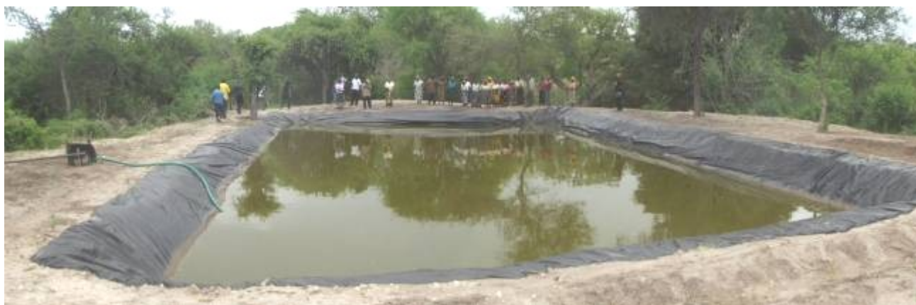
Photo 7: Community fishpond filled with water from a sand dam
