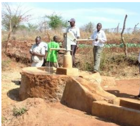
Photo 32: Shallow well with hand-pump and cattle trough, Kenya
