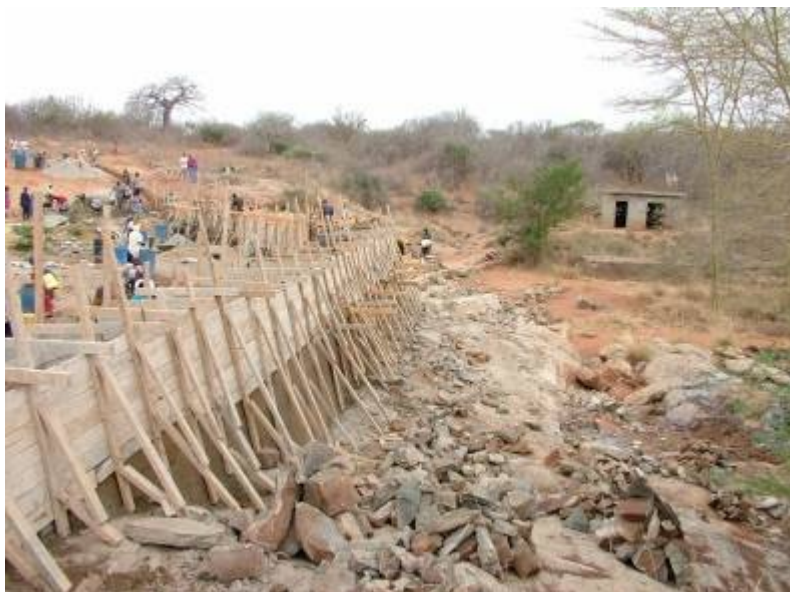
Photo 34: Formwork creates a mould for the stone masonry
