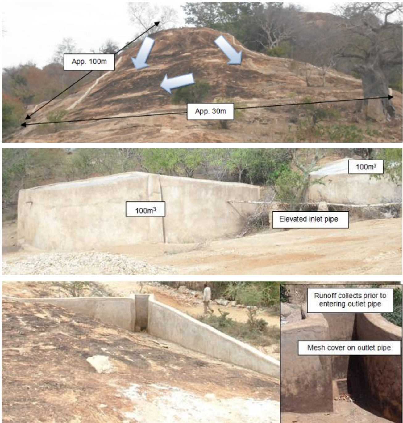
Photo 46: Rock catchment and storage tanks
