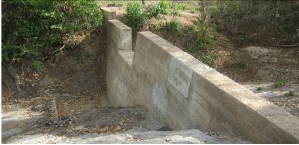
Photo 11: Dam 1, 250 bags of cement
