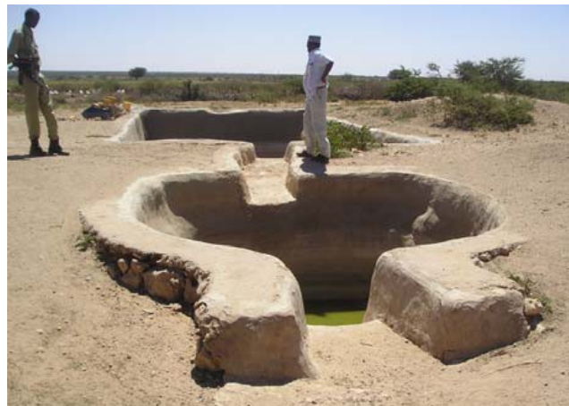
Photo 45: Run-off is channelled into a silt trap before entering the Berkad. Credit: Erik Nissen-Petersen
