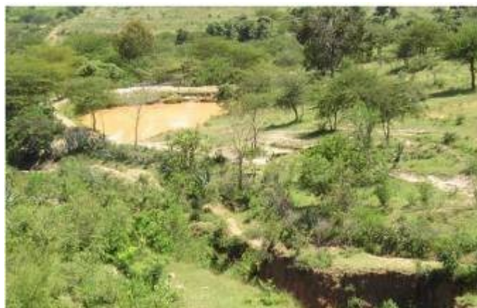
Photo 42: Hillside Dam, Kenya. Credit: E. Nissen-Petersen
