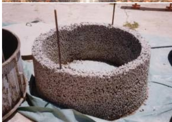
Photo 28: A no-fines concrete caisson Credit: Dabane Trust
