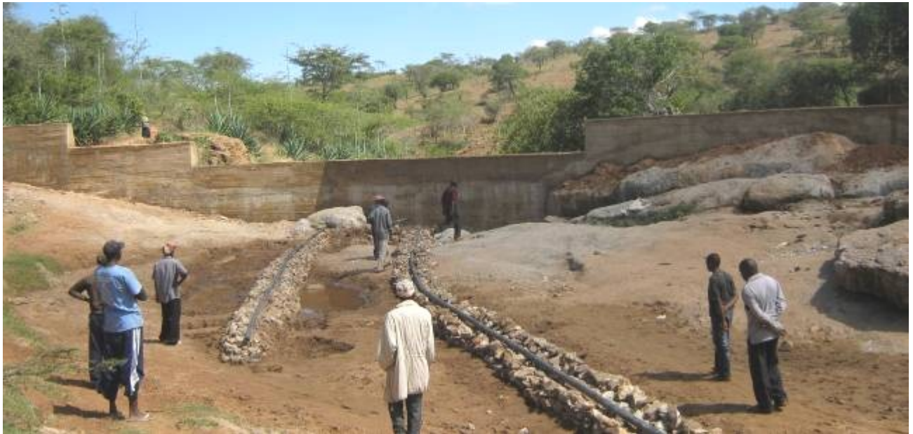
Photo 27: Installation of infiltration gallery
