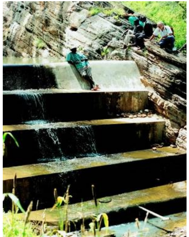
Photo 20: Stepped spillway: alternative method for progressive extension of central dam spillway
