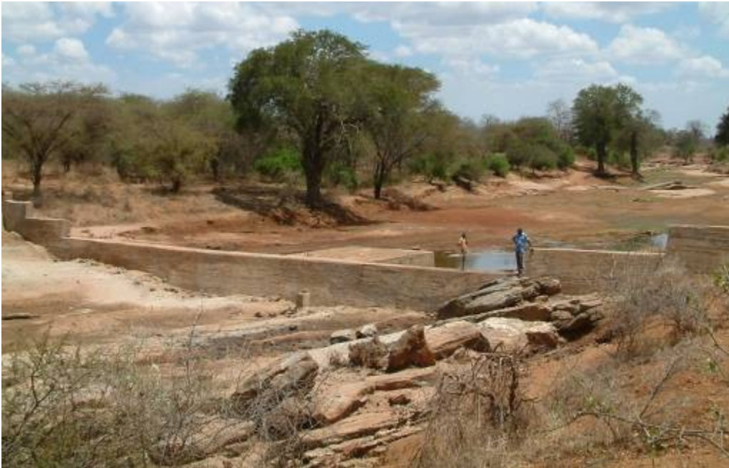
Photo 12: Dam 2, 810 bags of cement and 30 times more storage than dam 1
