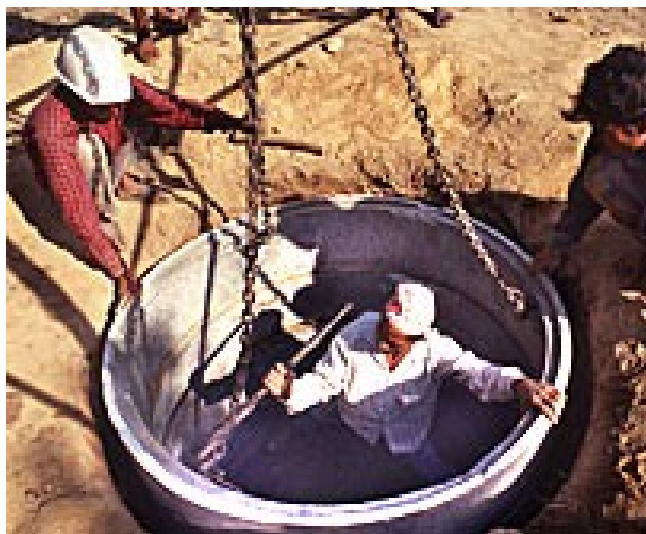
Photo 31: Safe excavation inside pre-cast concrete rings, Nepal. Credit: WaterAid / Caroline Penn
