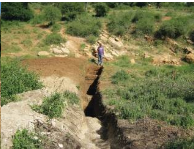
Photo 15: Test pits and probing confirm depth of bedrock
