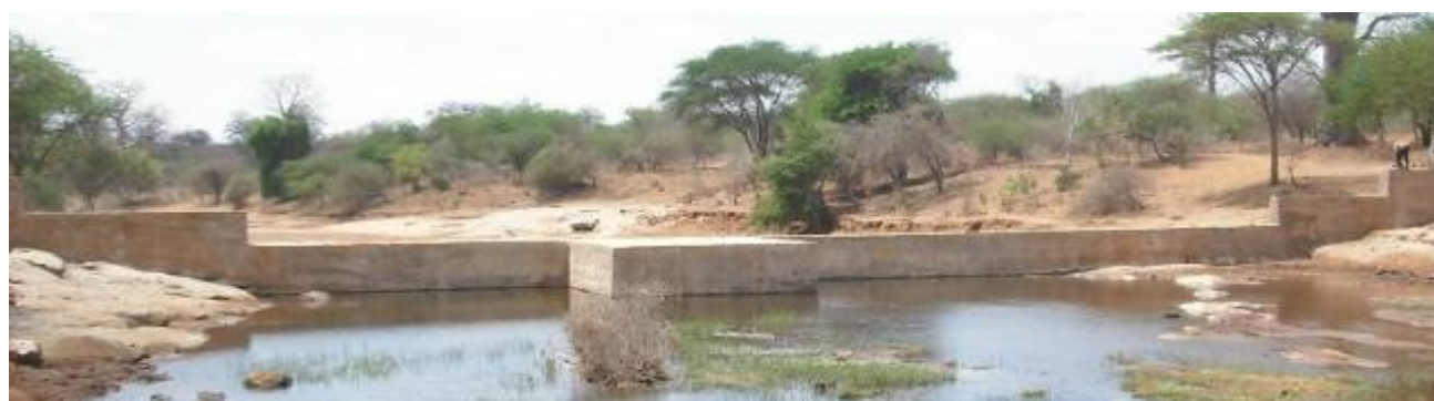
Photo 29: Tank built into wall of dam
