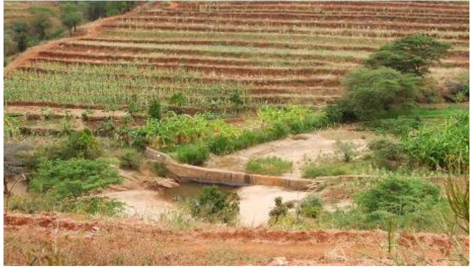
Photo 22: Terraces control runoff, increase infiltration and recharge and reduce gulley formation and erosion around the wings
