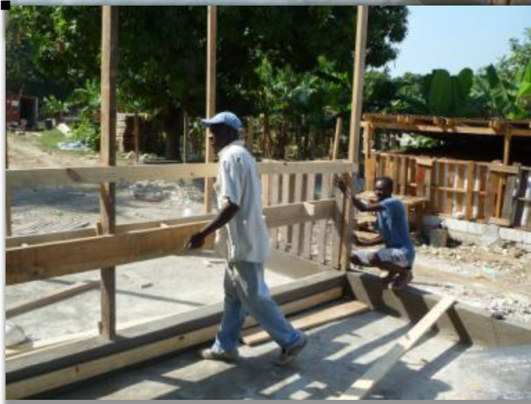
Photo K112: Interior walls construction.
