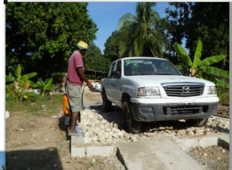
Photo K218a,b: Chlorine spray station for vehicles
