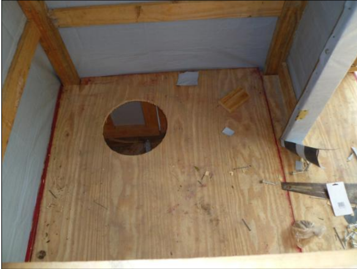
PHOTO T5: Poophole cut in plywood floor
