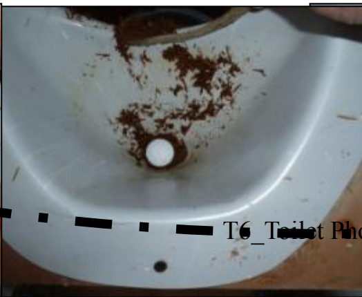
PHOTO T17 Unclogging urine bowl in UD seat
