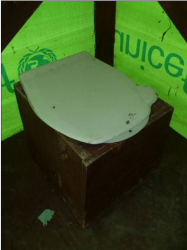
PHOTO T13a: SOIL UD toilet seat, view on outside
