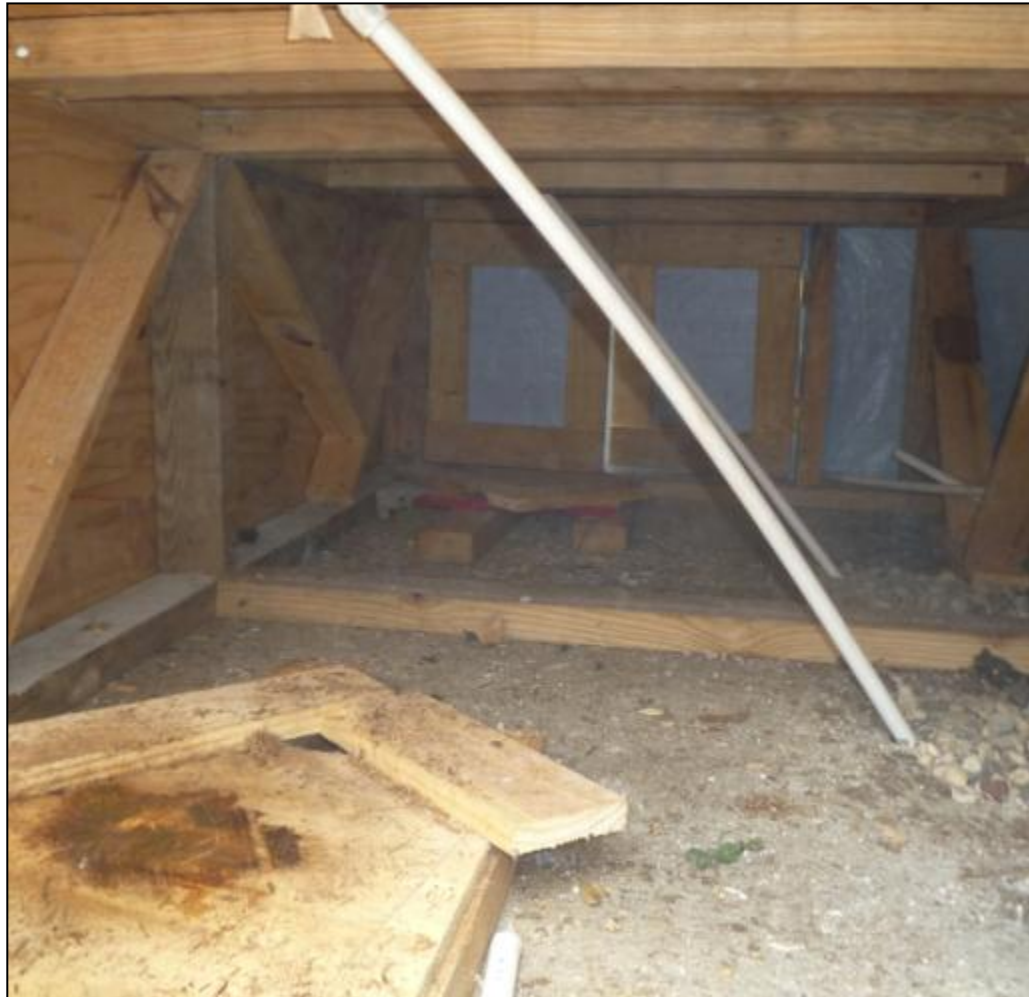
PHOTO T1: Chamber beneath toilet
