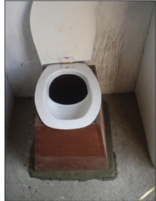
PHOTO T13c: SOIL UD toilet seat, view on outside
