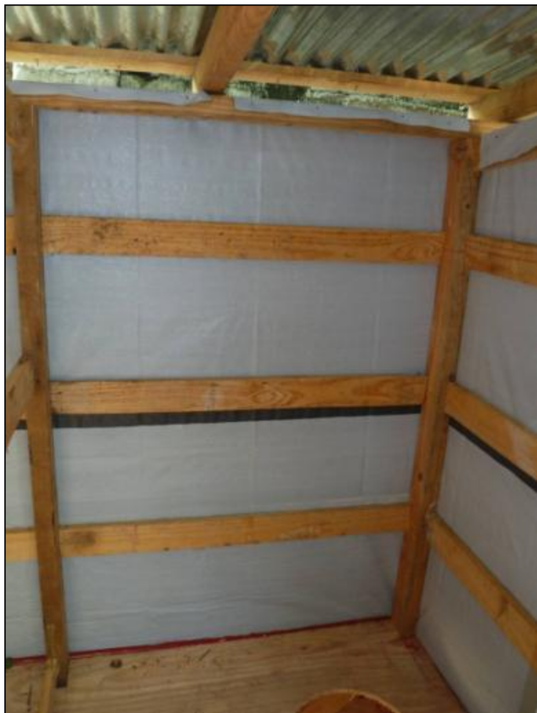
PHOTO T9: Internal Walls
