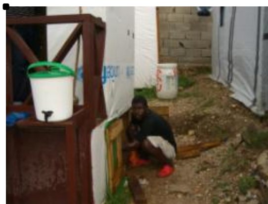
A toilet operator moves a clean empty drum into a SOIL UD toilet.
