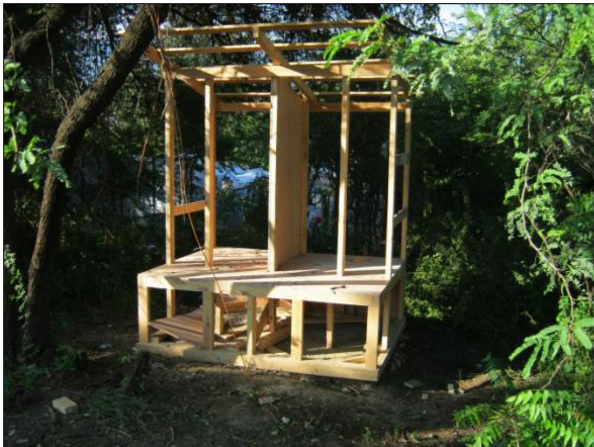
PHOTO T10: Wooden Structure
