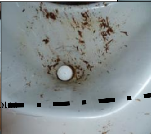
PHOTO T17 Unclogging urine bowl in UD seat
