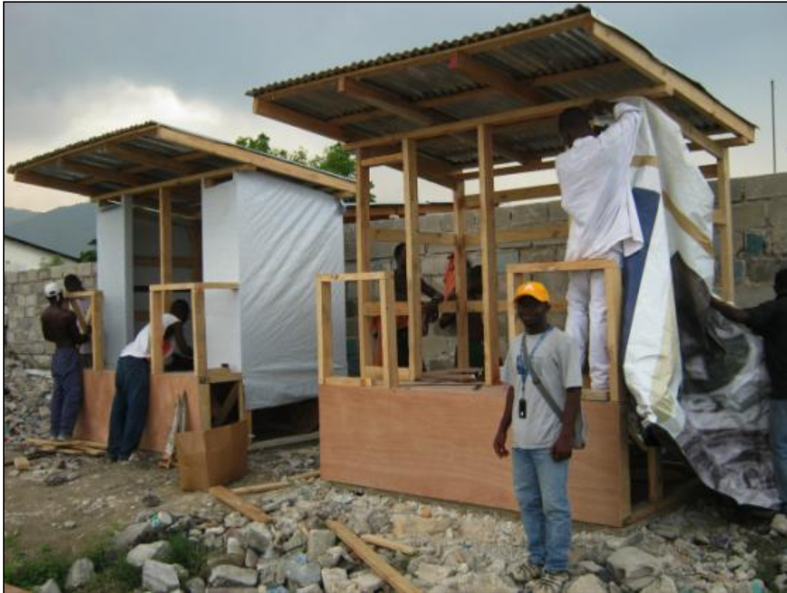
PHOTO T7: Plastic Sheeting cladding on wooden structure
