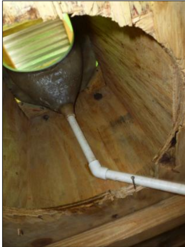
PHOTO T13b: SOIL UD toilet seat, view from poophole
