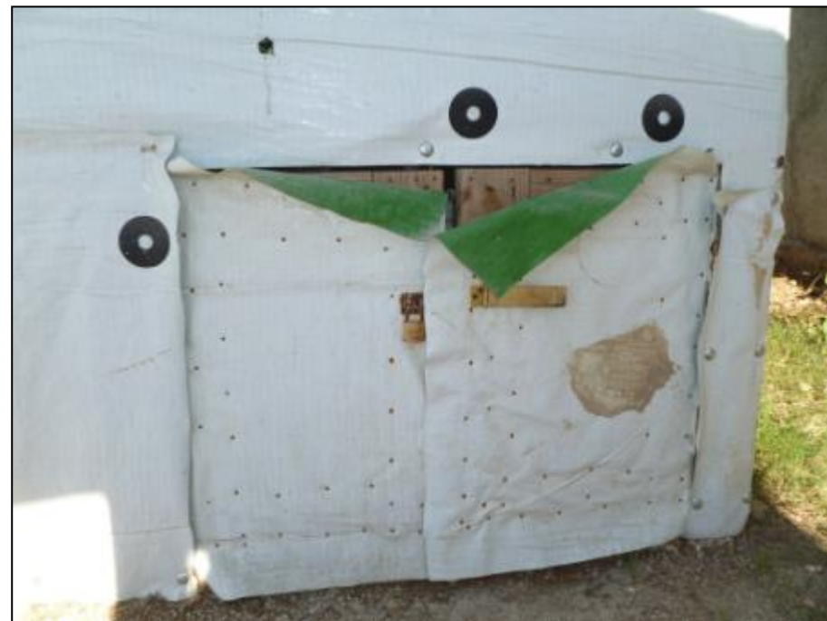
PHOTO T12: Close-up on chamber doors
